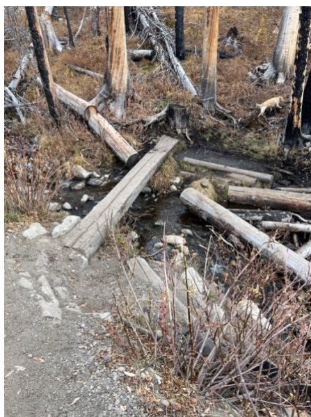
Water crossing at .81 miles
