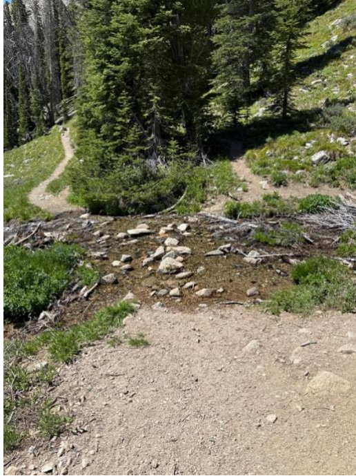
Stream crossing at about 3.6 miles
