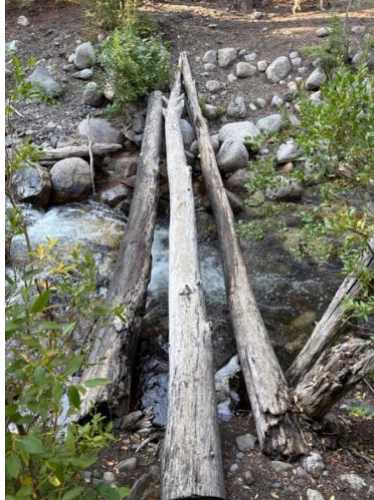
Creek crossing at 1.8 miles
